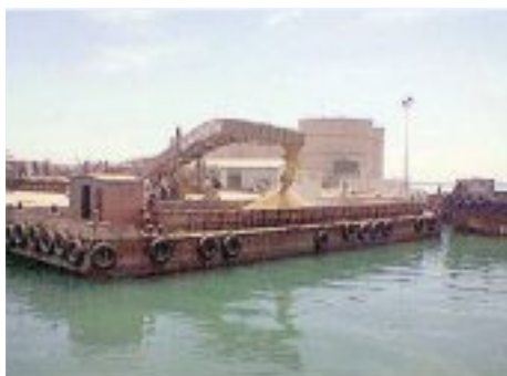
Mobile barge loading system with capacity of 450 TPH at Ruchi Soya jetty, Jamnagar installed on build, own and operate (BOO) basis.
