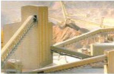
Bulk Material Handling system at a mine site
