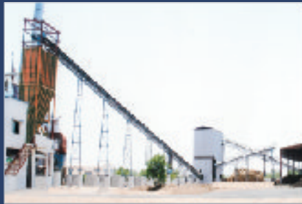
▲ Coal Handling System.
