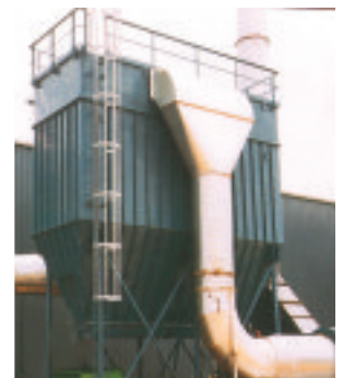
Pulse jet type bag filter
