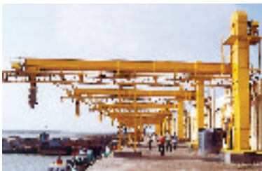
1000 TPH Barge loading infrastructure at Bedi Port, Jamnagar.
