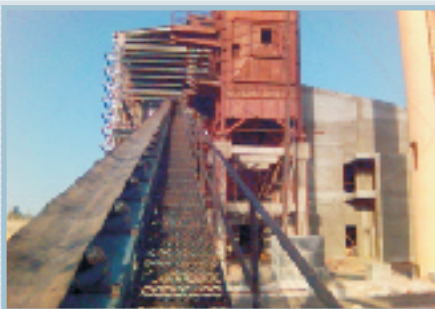
Belt conveyor under erection
