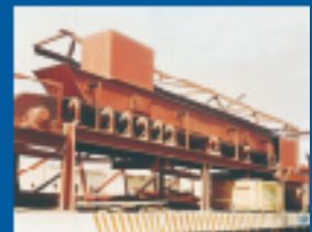
Belt conveyor for conveying iron ore-part at alloy steel addition system.
