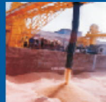
Telescopic chute discharging DOC at port site.
