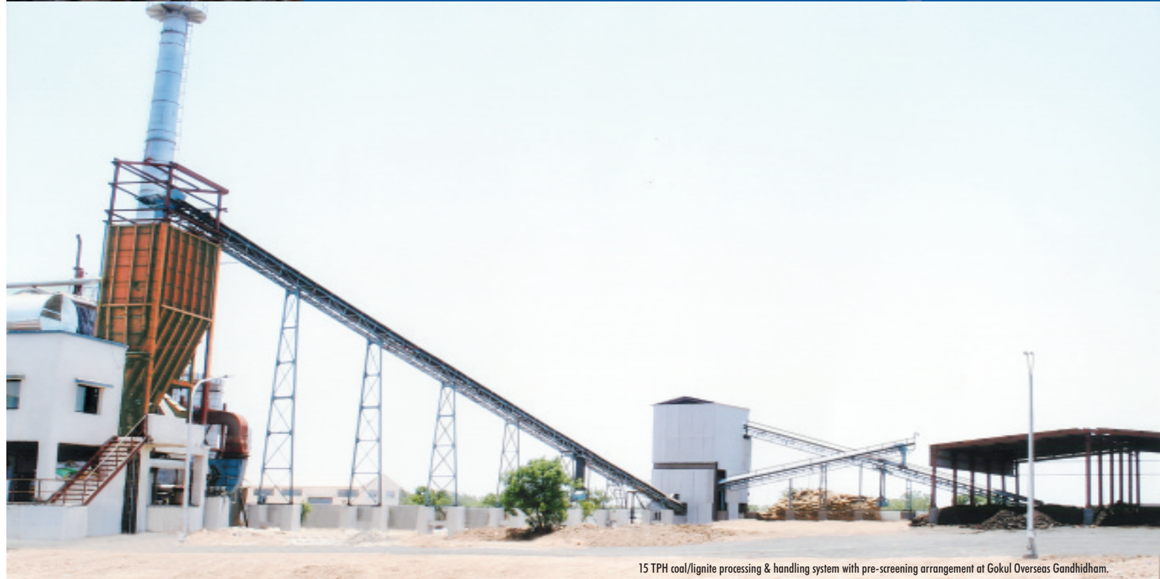
15 TPH coal/lignite processing & handling system with pre-screening arrangement at Gokul Overseas Gandhidham.
