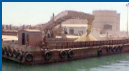
Mobile barge loading system with capacity of 450 TPH at Ruchi Soya jetty, Jamnagar.
