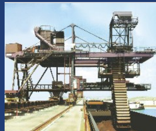
Barge Unloading System
